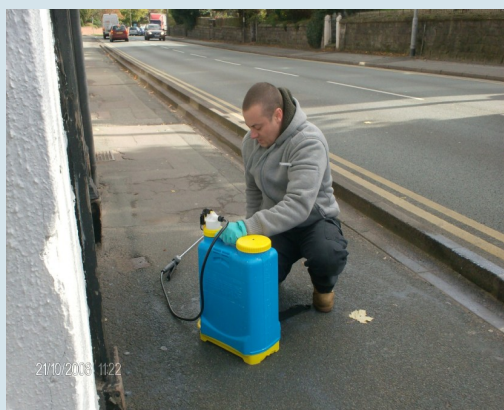
Photo: application of Photo-catalytic paint (left) and the area sprayed (Right) in West Road, Congleton
